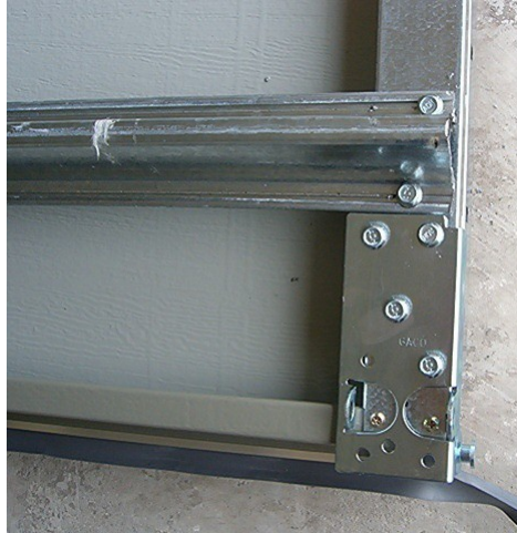
Figure 1A – Bracket & Strut Position on Bottom Panel
