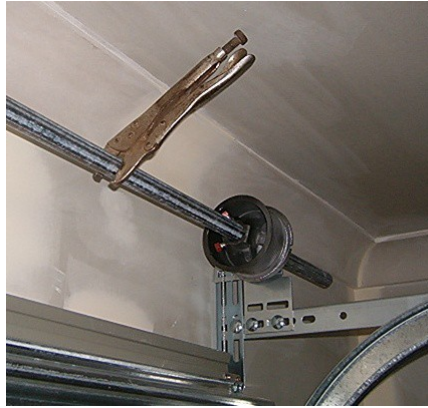
Figure 10 – Clamping Shaft Prior to Spring Tensioning (vice-grips resting against ceiling in this case)
