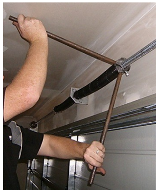
Figure 11 – Tensioning Springs
