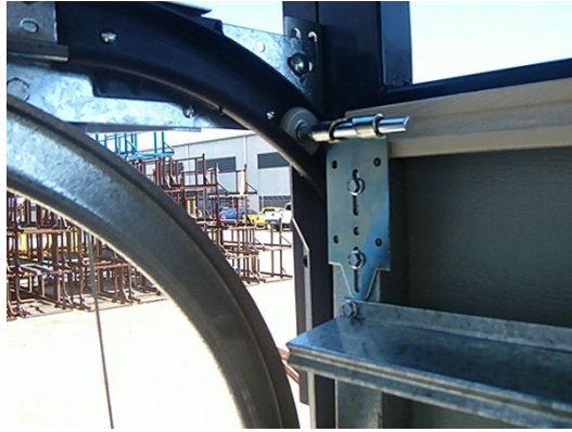
Figure 9 – LHR Top Bracket Mounting
